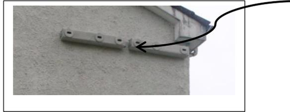
The tweeter is located outside as near to the boxes as possible, as described above. The amplifier (with or without timer) should be located **inside** a building or in a protective box so that it is not exposed to the weather.
